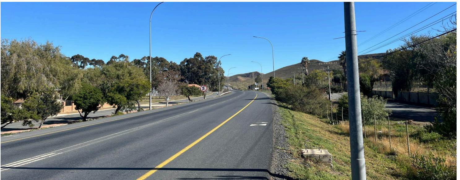
Figure 4.6: Facing west, towards the entrance of Laingsburg
