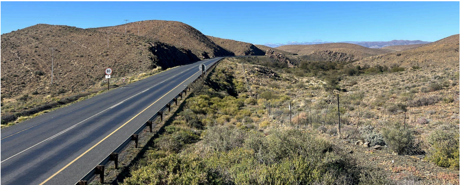
Figure 4.8: Facing east, towards a part of the route that cuts through the bedrock area.
