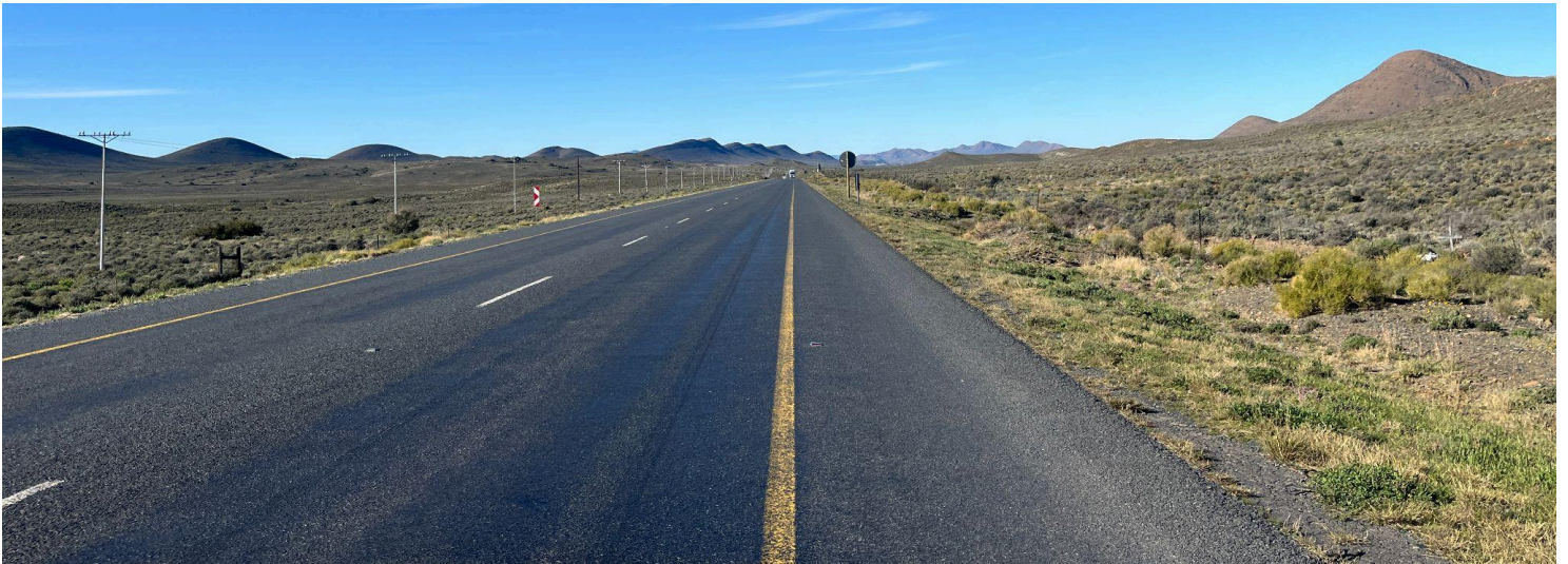
Figure 4.19: Facing east, near the western end of the proposed upgrades
