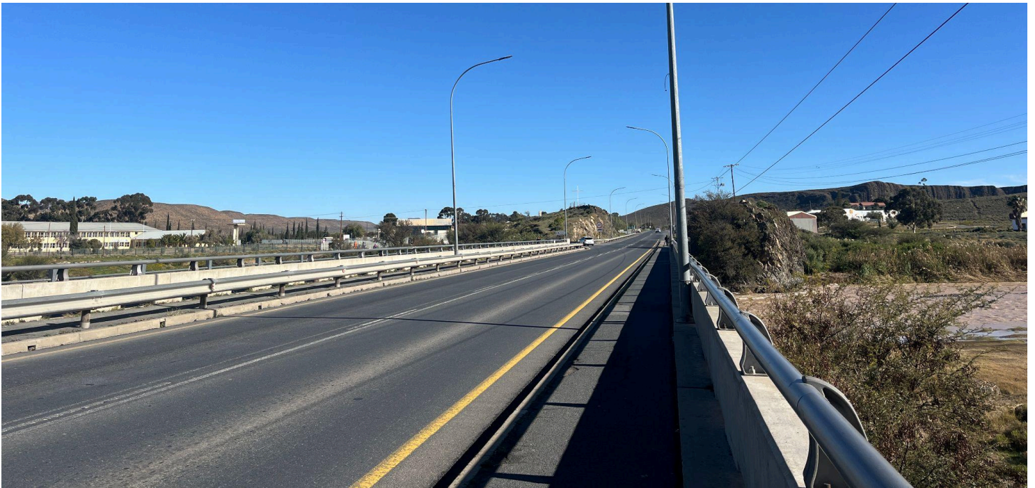
Figure 4.3: The bridge that crosses the Buffelsrivier
