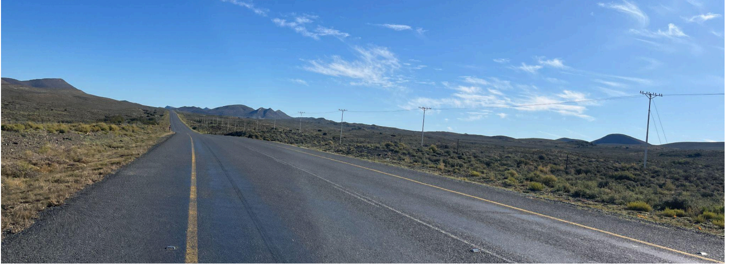
Figure 4.18: Facing west, near the western end of the proposed upgrades
